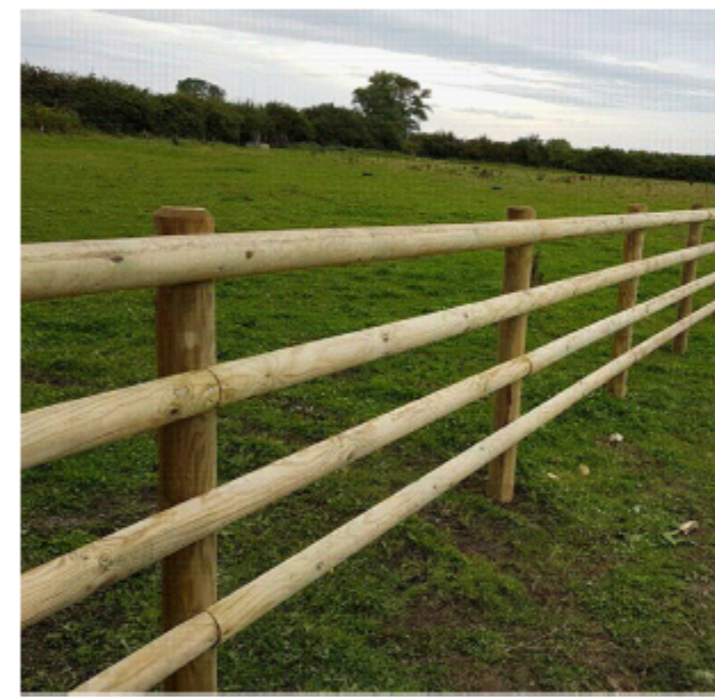
Detail B - Proposed Timber Post and 4 Rail Fence (or similar approved)
